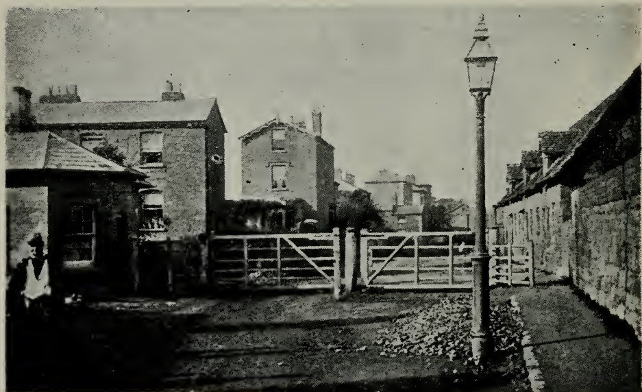
ABOVE EIGN TURNPIKE GATE. ABOLISHED 1870
